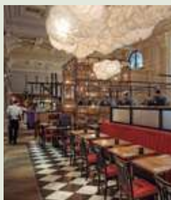
Burger & Lobster restaurant. Bath, UK. Panasonic's air-to-water Aquarea system has been installed in the latest glamorous Burger & Lobster restaurant in Bath. The Octagon Chapel, a large listed building in the city centre, was converted to accommodate the restaurant, and Panasonic's Aquarea system provided an extensive, energy efficient and unobtrusive heating and cooling solution.
