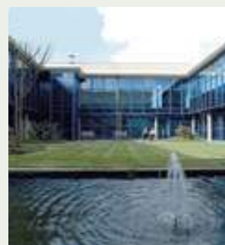
NHS Canford house clinic, Bournemouth, UK. VRF
