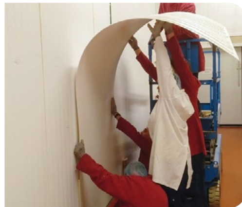
Installation of FRP sheet 2 mm Smooth.
