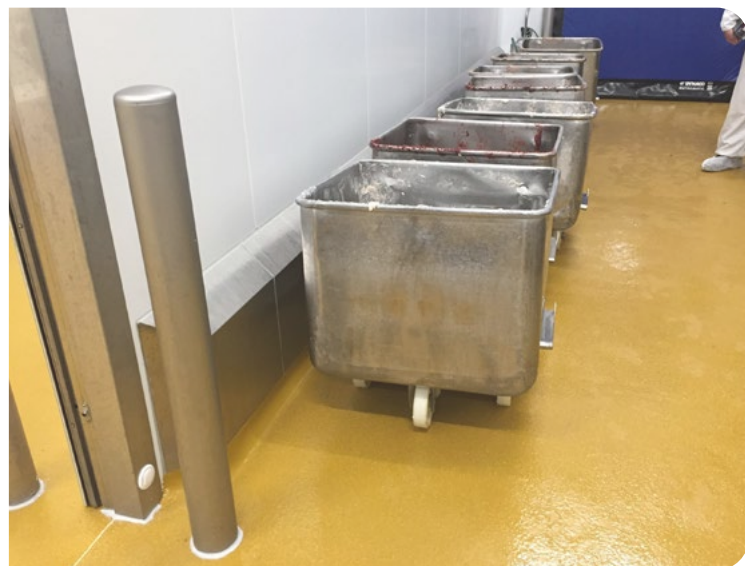
PolySto prefabricated ICS40RB stainless steel kerb with concrete core with a resin floor applied into the rebate.
