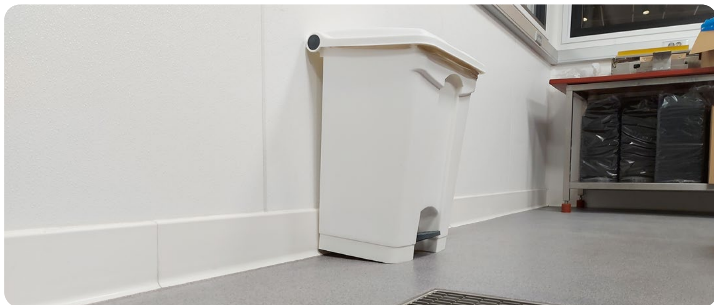
PolySto prefabricated PV15F full core PVC skirting installed against a FRP embossed sheet, finished with HygiSeal.
