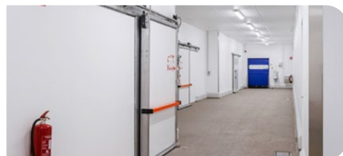
FRP HygiWall in a ready meal facility.
