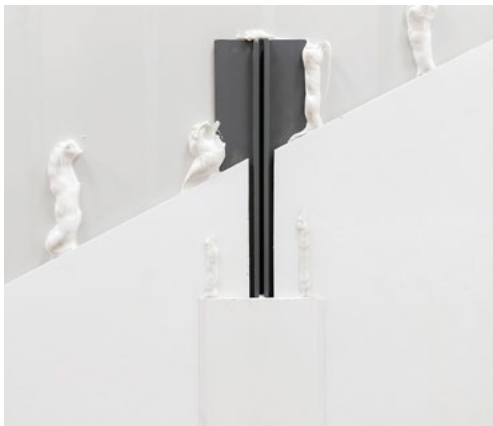
FRP sheets finished with PVC profiles.
