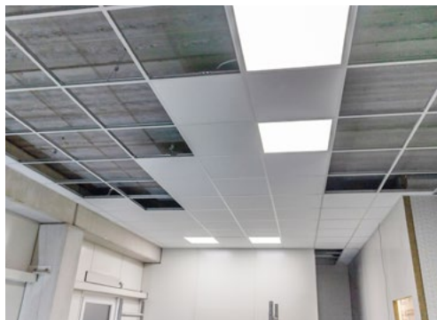
Installation of FRP HygiCeiling.
