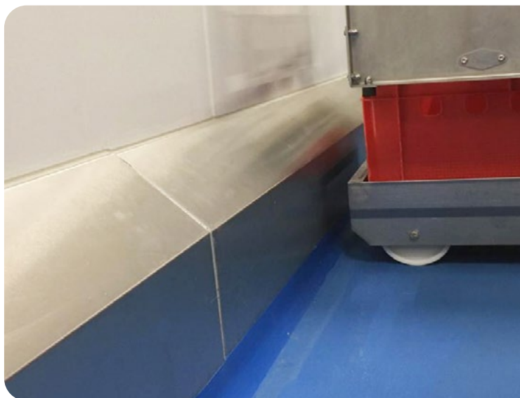
PolySto prefabricated ICS40RB stainless steel kerb with concrete core with a resin floor applied into the rebate.
