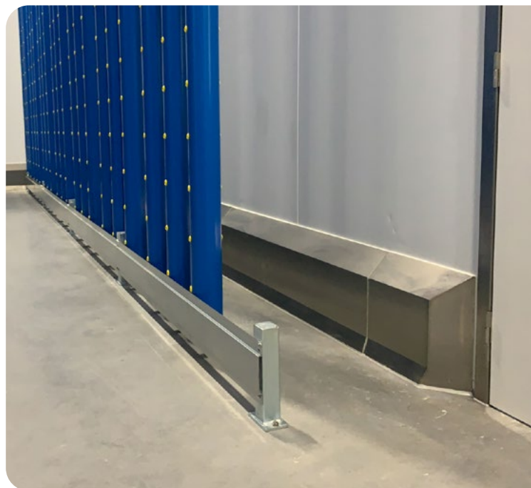
PolySto prefabricated ICS30F (left) and OCS30F (right) stainless steel kerb with concrete core installed on top of a concrete or cast floor.
