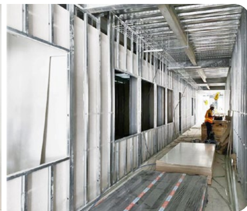
FRP RenoCemPanels can be installed on metal studs.
