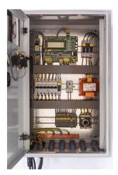
Metal casing painted with RAL7035, 120 micron thickness, suitable for outdoors installation.
