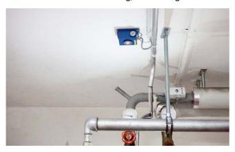
are designed for zone 1 or zone 2. The BUS mounted CWED 68 programmable sounder beacon with display or the Touch Screen displays can be installed at the entrance to the heating plant room allowing for easy viewing of the ambient gas levels with colour coded bar graphs to facilitate easy viewing of the gas monitoring status. All measurement data and alarm events are recorded.
