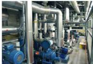
Refrigeration systems Typical gases: NH3, CO2, HFKW/HFCKW
