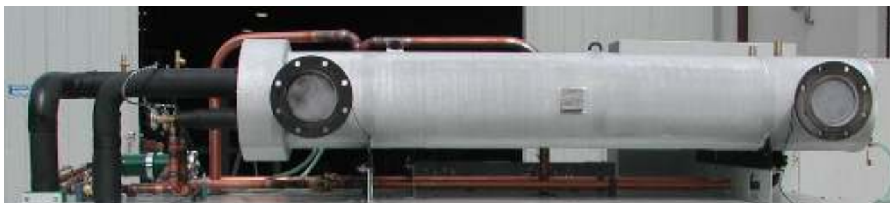
Evaporatore fascio tubiero - Shell and tube evaporator
